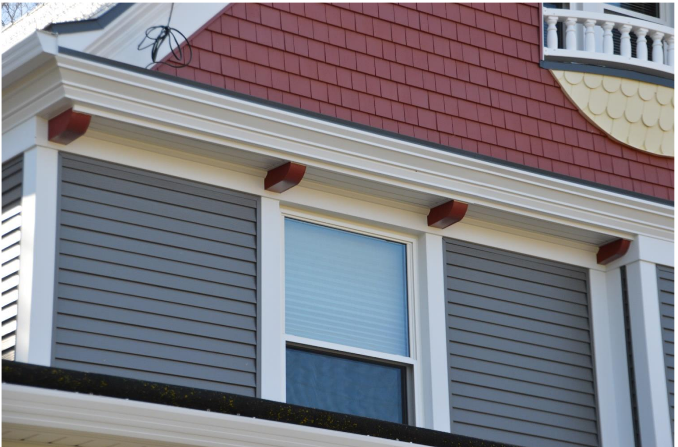
After--detail of corbels, now maintenance free
