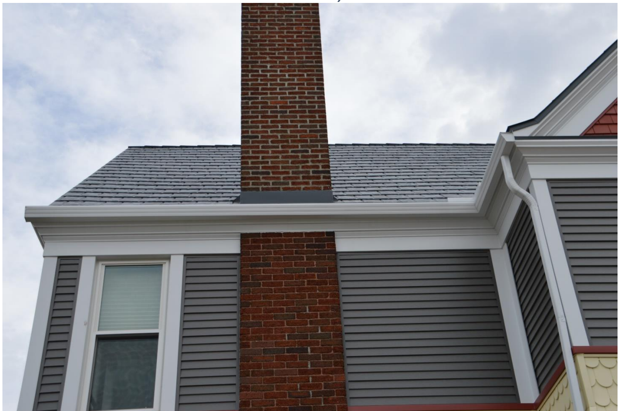
After : the re-configured roof edge accommodates the seamless gutter system, yet allows visibility of crown detail.
