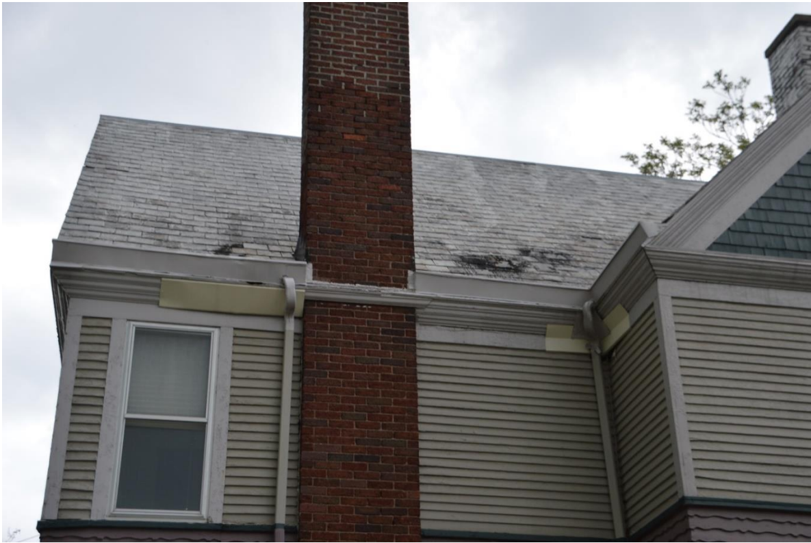
Before: Gutter system was an eyesore: poor placement of downspouts & did not continue across chimney area.
