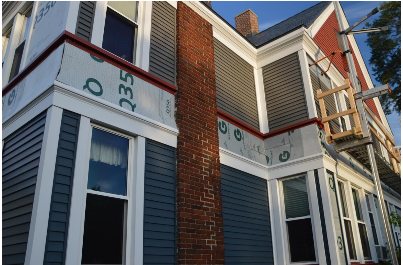
In progress-- renovating west wall area
