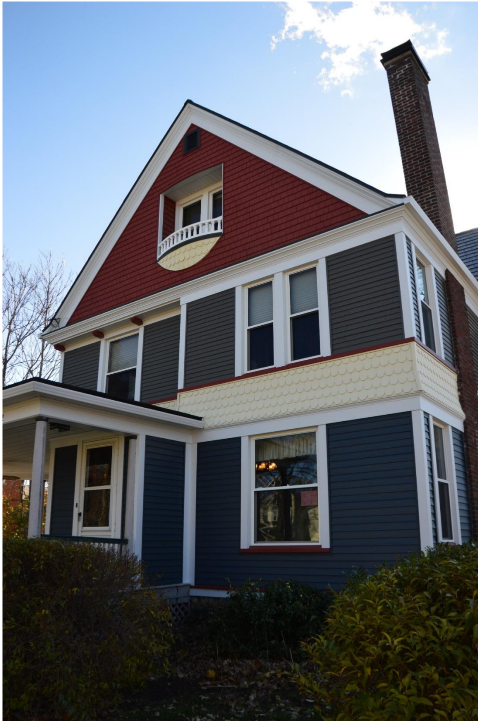
From top: ABC Seamless Glacier White trim, Mastic Perfection T-5 Shake in Russet Red, Mastic half round shake in Almond, ABC Seamless in Charcoal Gray T-3 & Classic Blue T-4 straight.
