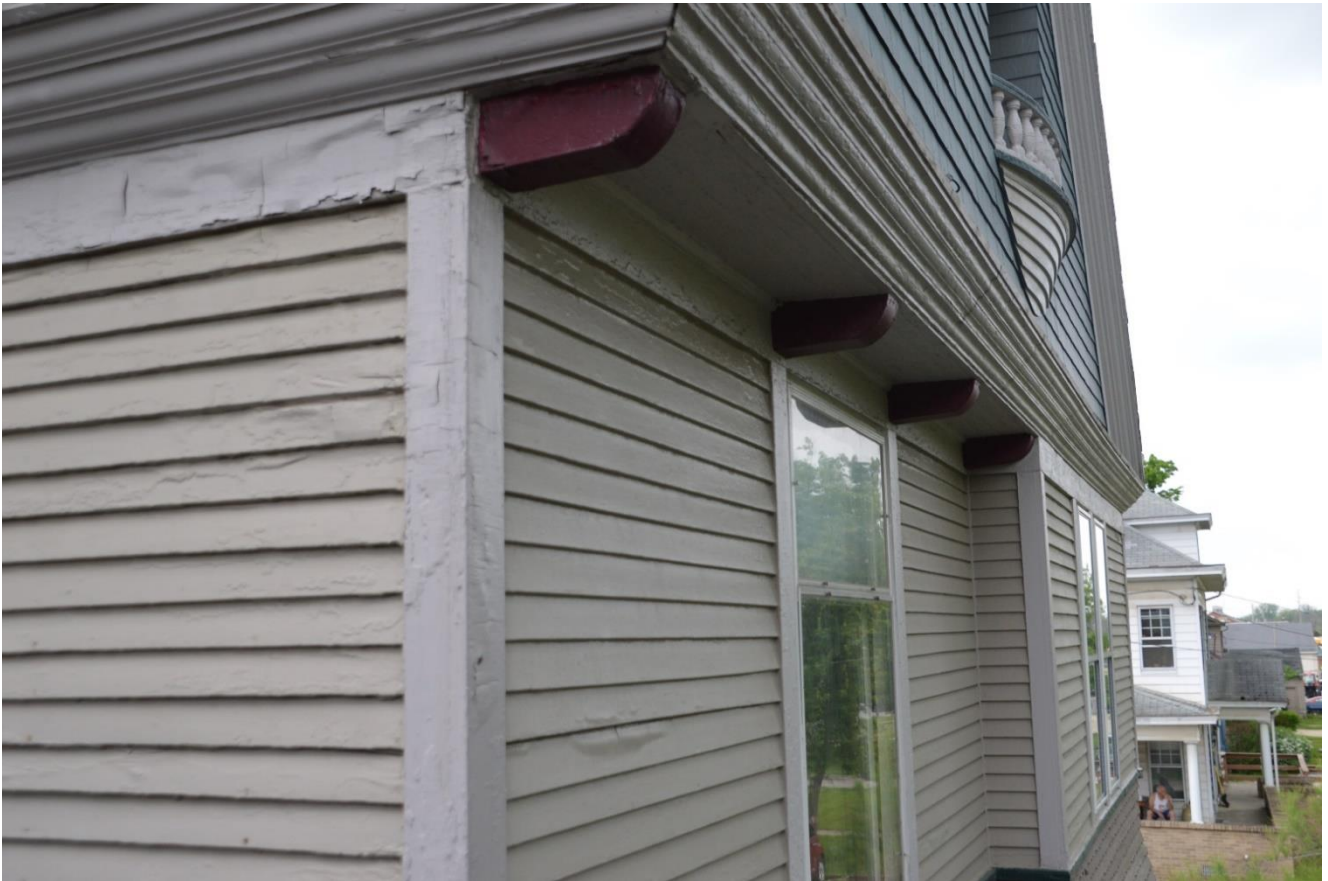
Before--detail of corbels
