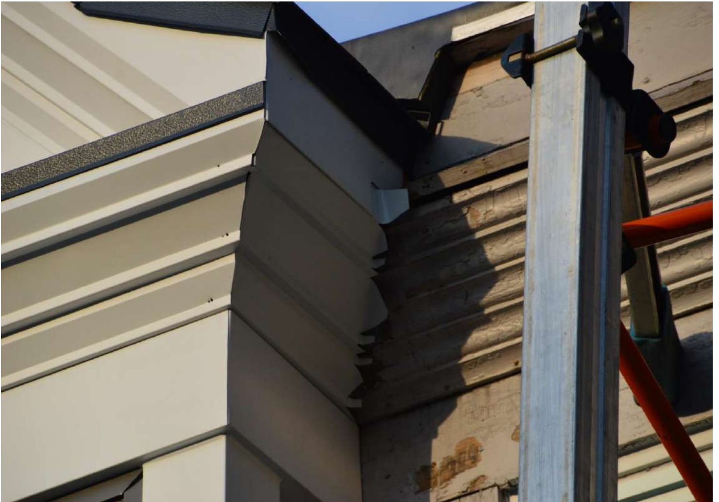
In progress: Detail of how a single piece of trim was bent and carefully cut to recreate the multi-tiered crown with 30 gauge steel.
