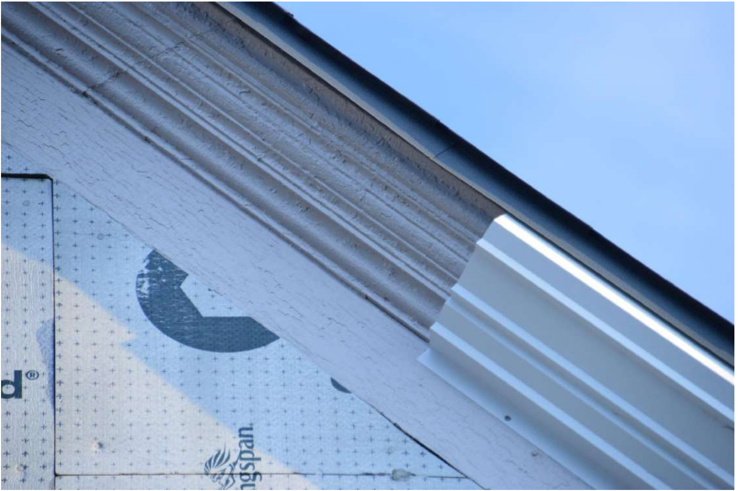
In process; replicating rake edge trim
