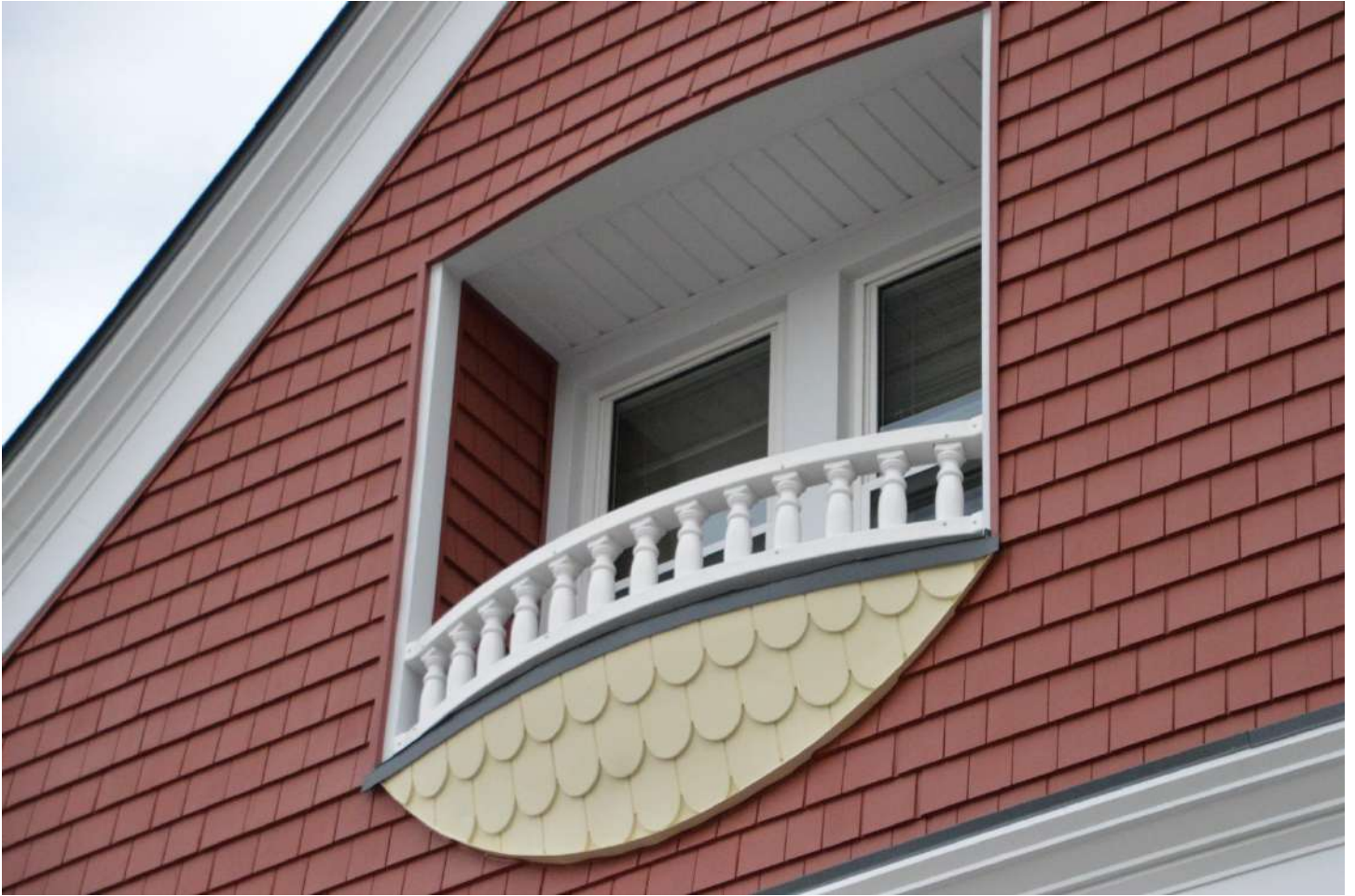
After: Custom-formed radius for vinyl rail that replaced a wooden one.
