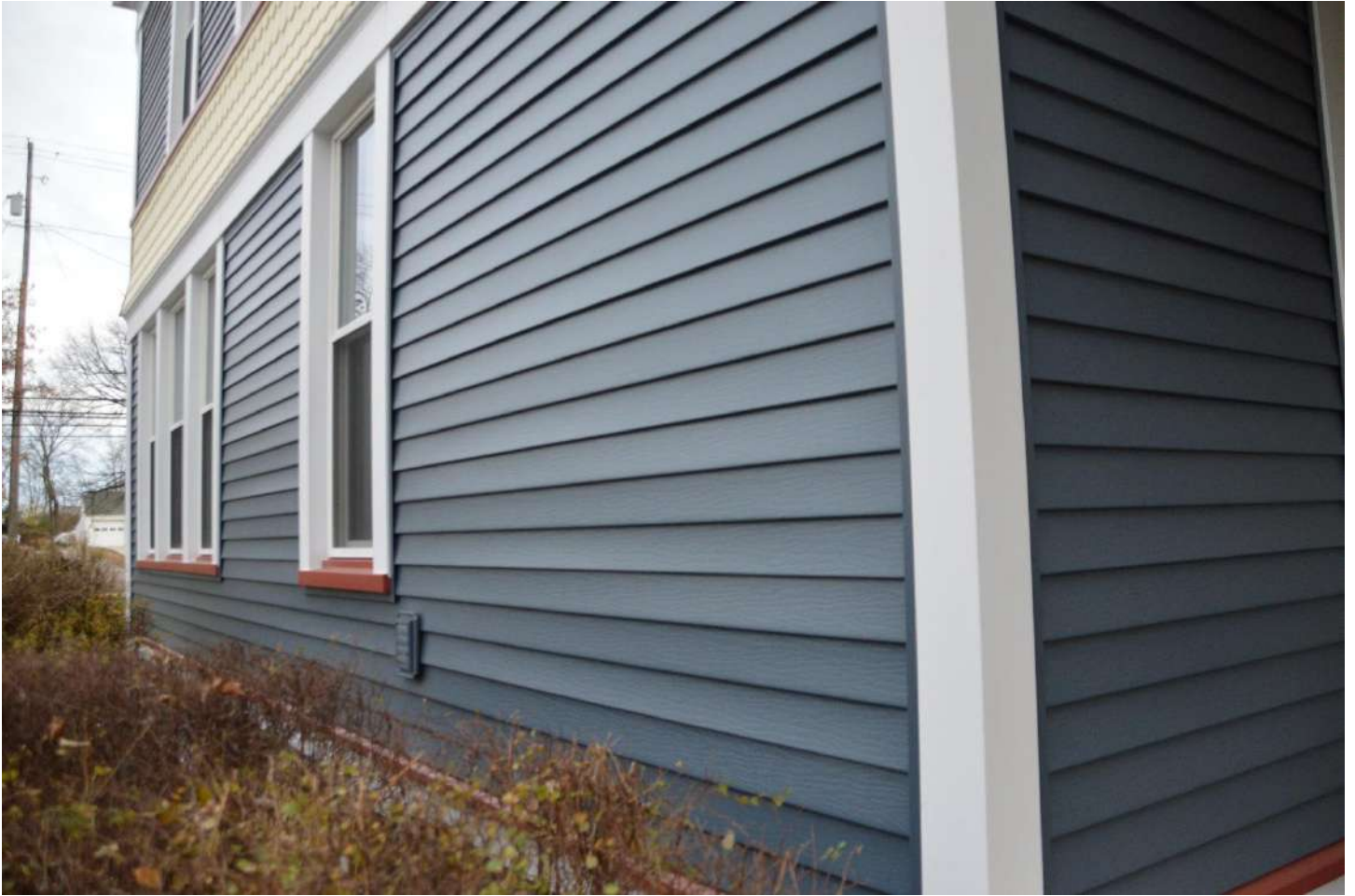
ABC Seamless steel siding provides a clapboard siding appearance for this 1906, Queen Anne style home
