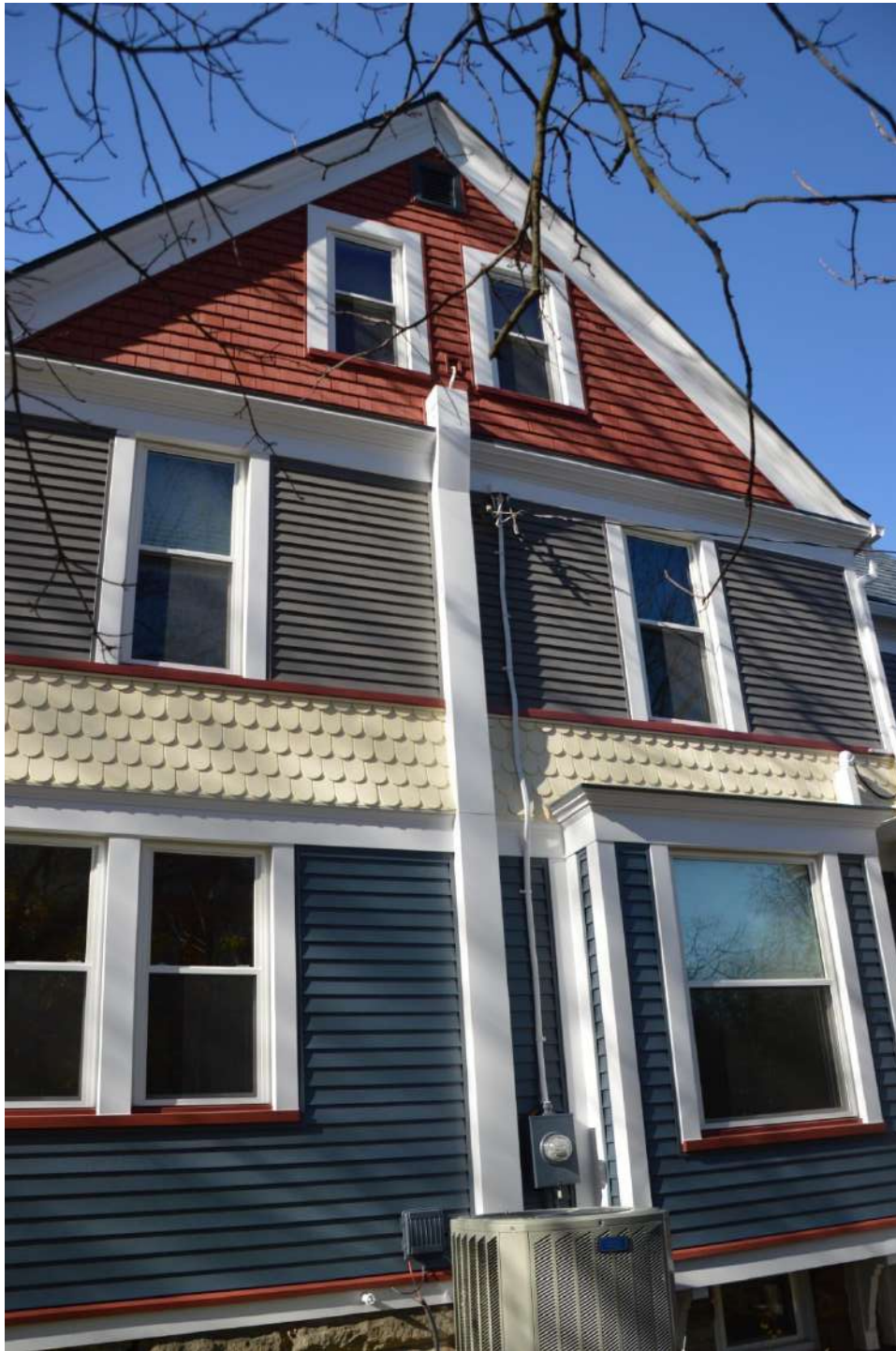
By creating custom chase covers, the non-electric utility cables where hidden.
